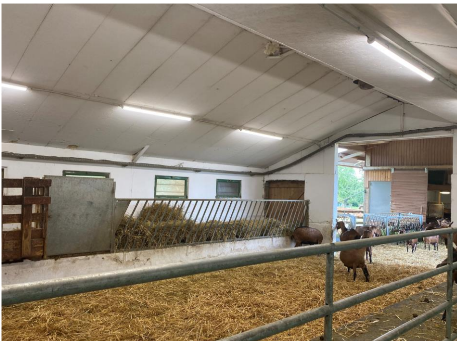
Bright light in the goat stall through the new DAMP PROOF SPECIAL luminaires.
