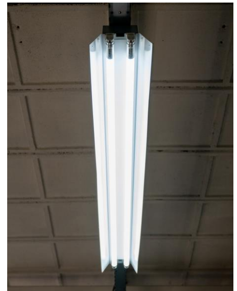
T8 EM PRO ULTRA OUTPUT LED tube directly connected to the 230V mains.
