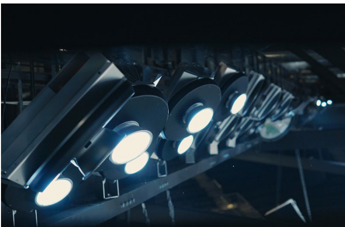
Each floodlight features two optical modules, allowing for precise control over lighting intensity
