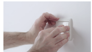
04 Mount the cover of the pushbutton.
